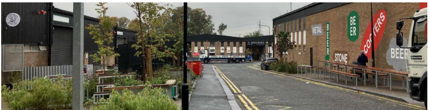
Figure 15: An elevation of a unit at Lockwood Way Industrial Estate, illustrating the public realm interventions (Source: We Made That)
