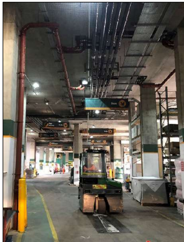
Figure 10: Within the completed Travis Perkins scheme, the number and location of internal columns and shelves has created practical challenges for the movement of vehicles within the internal space. (Source: Deloitte)
